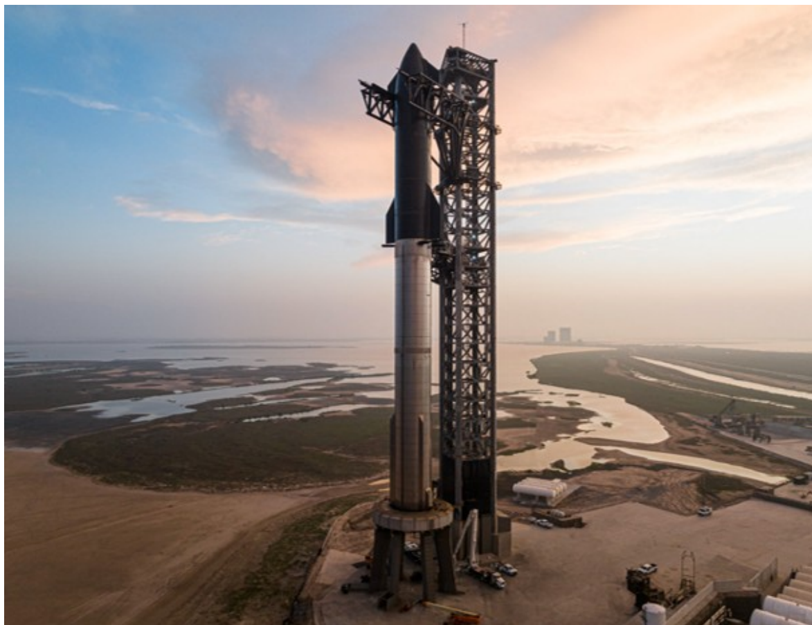
Fig. 12 Block 1 version of SpaceX super heavy launch vehicle on launch pad in Starbase, Texas
